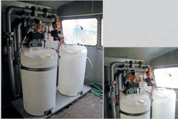
Fig. 3 – Example of injection unit (Photo: Photo: A. Godyń).
